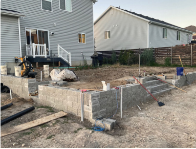
Walker's backyard in the renovation process
